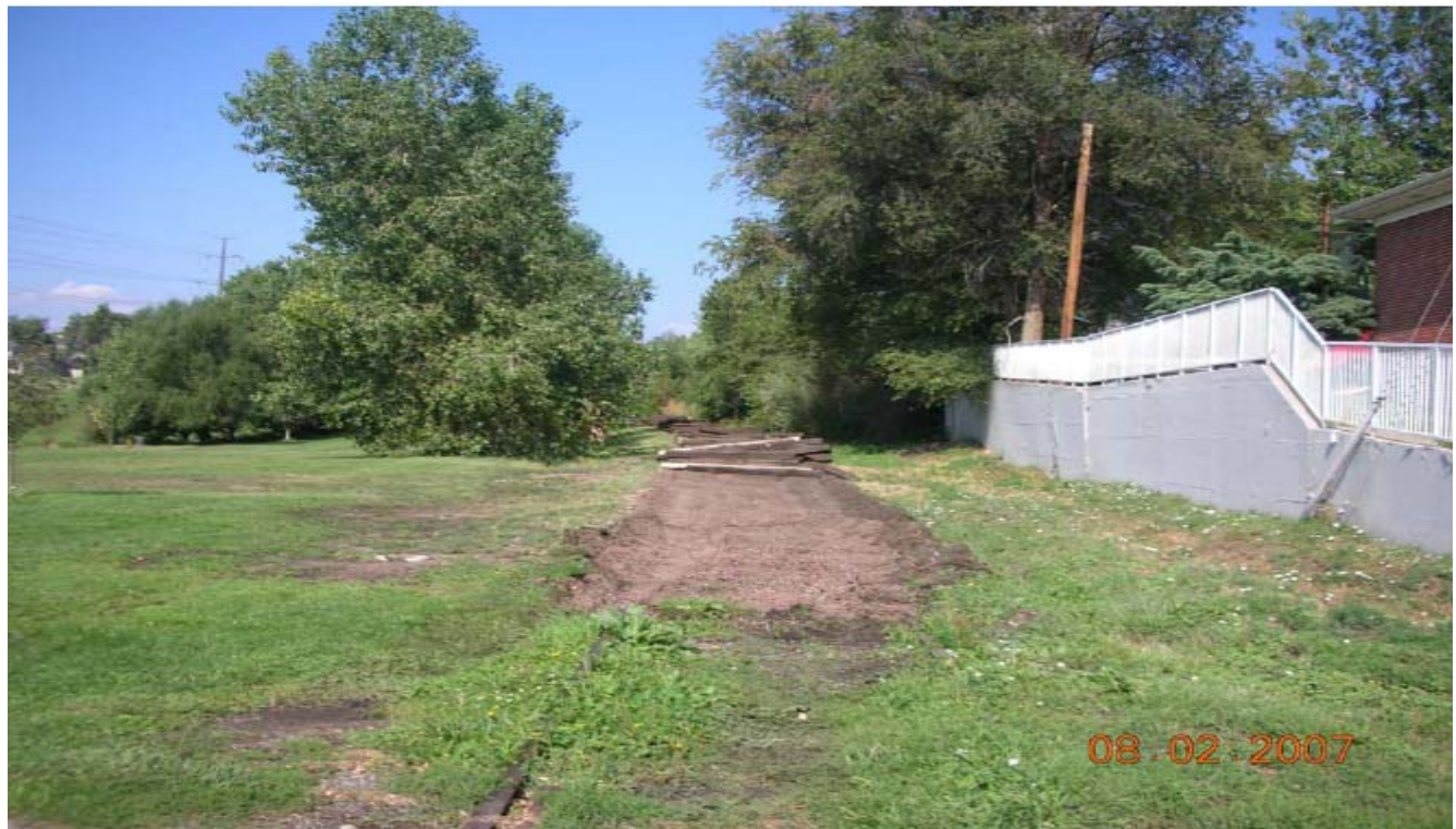
Ties staged for processing immediately west of Knox Ct. (1566+50)
