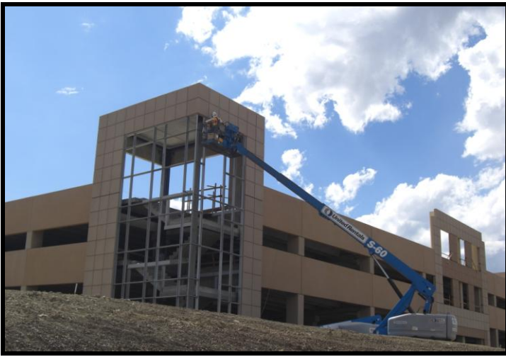
Jeffco Parking Structure - August 2011
