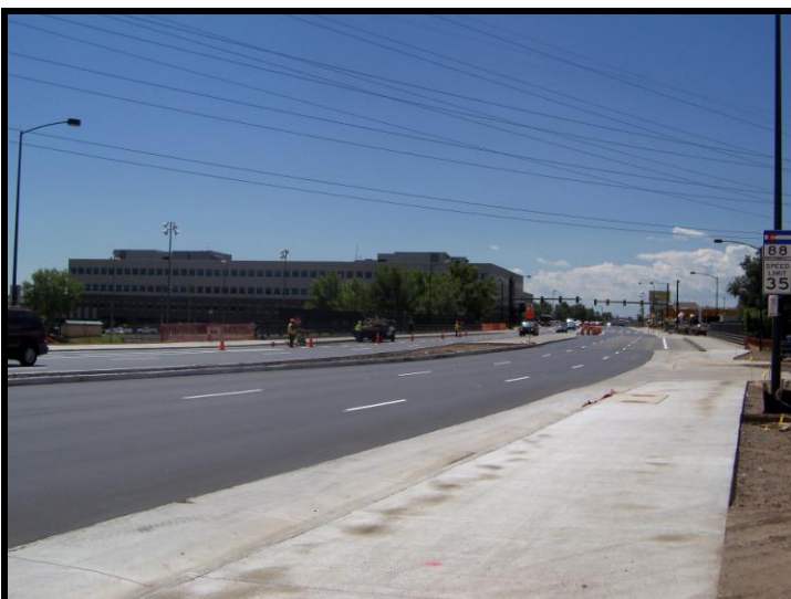
Federal Boulevard Bridge- August 2011
