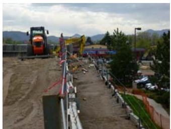
Wadsworth Bike Bridge Construction
