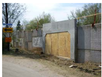
Wadsworth Bike Bridge Construction
