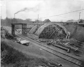
Construction of the Federal Bridge- 1922
