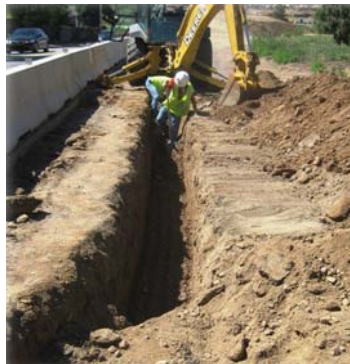
Crews work to relocate a gas line near Sheridan Boulevard
