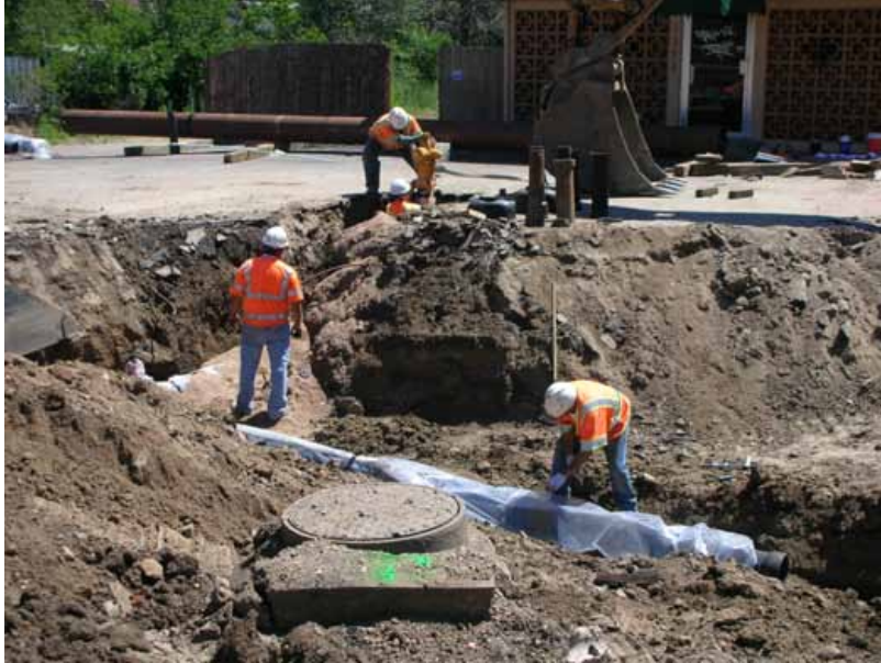
Fire Hydrant Installation Crews work to install a fire hydrant above.
