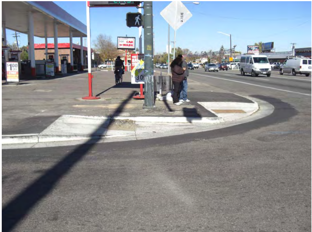
Curb and gutter work at 14th and Sheridan
