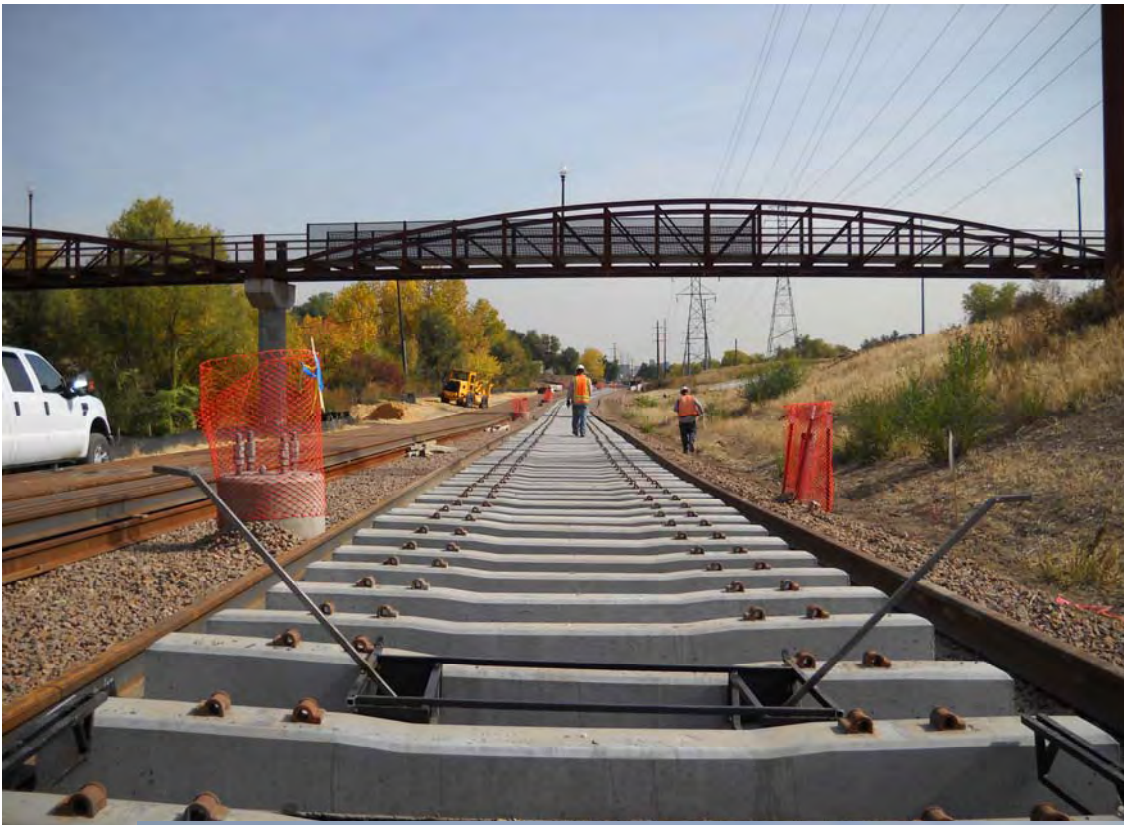
Skeleton Track installation—Sheridan to Perry
