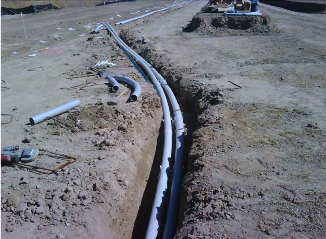
Ductbank Installation between 6th Avenue and Union
