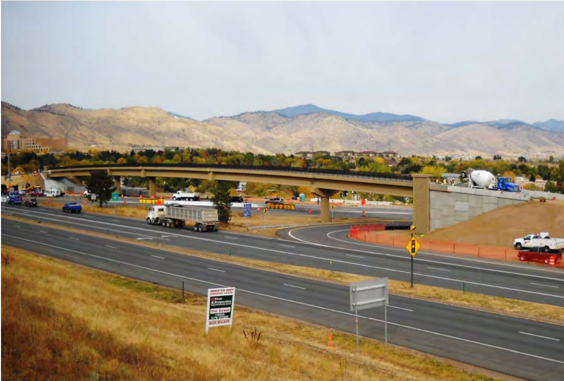
Colfax Bridge Approach walls and final paint
