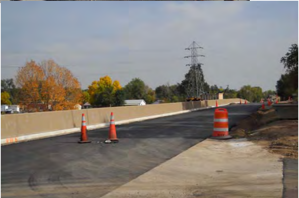
Roadway Paving on 13th Avenue at Carr
