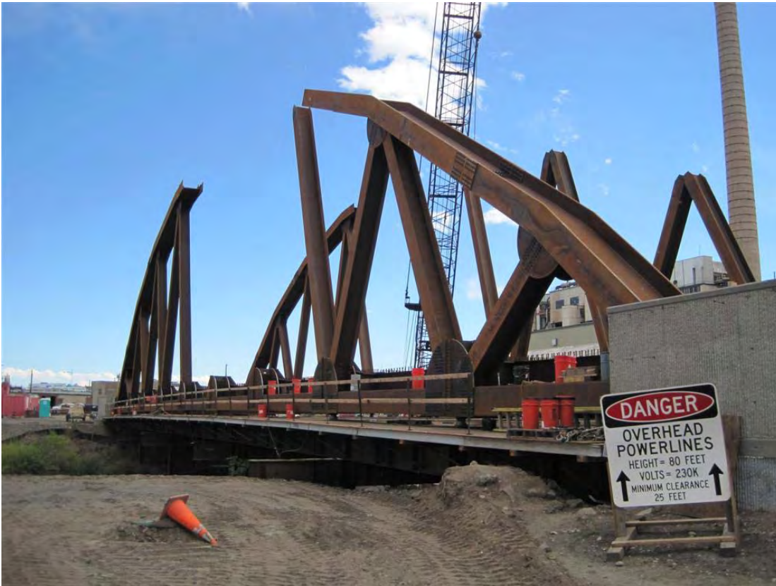
South Platte River Bridge Assembly
