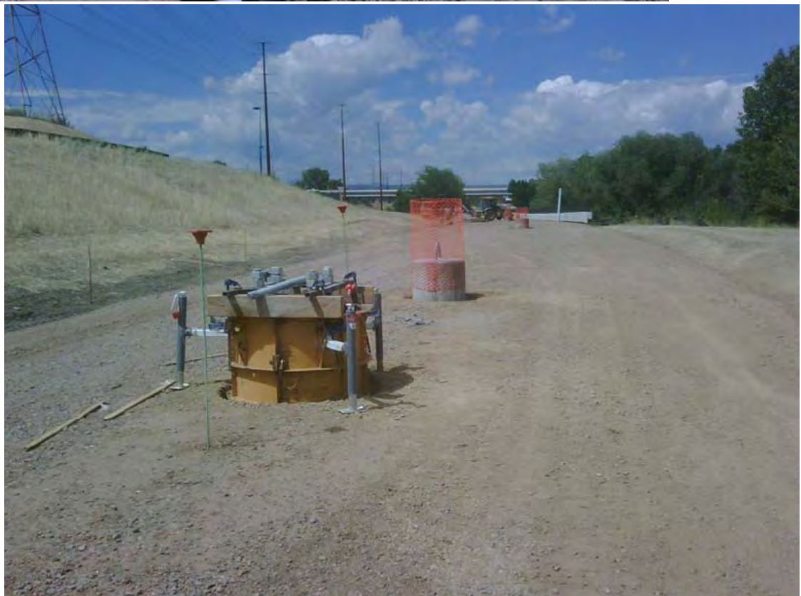
Overhead catenary system foun- dations
