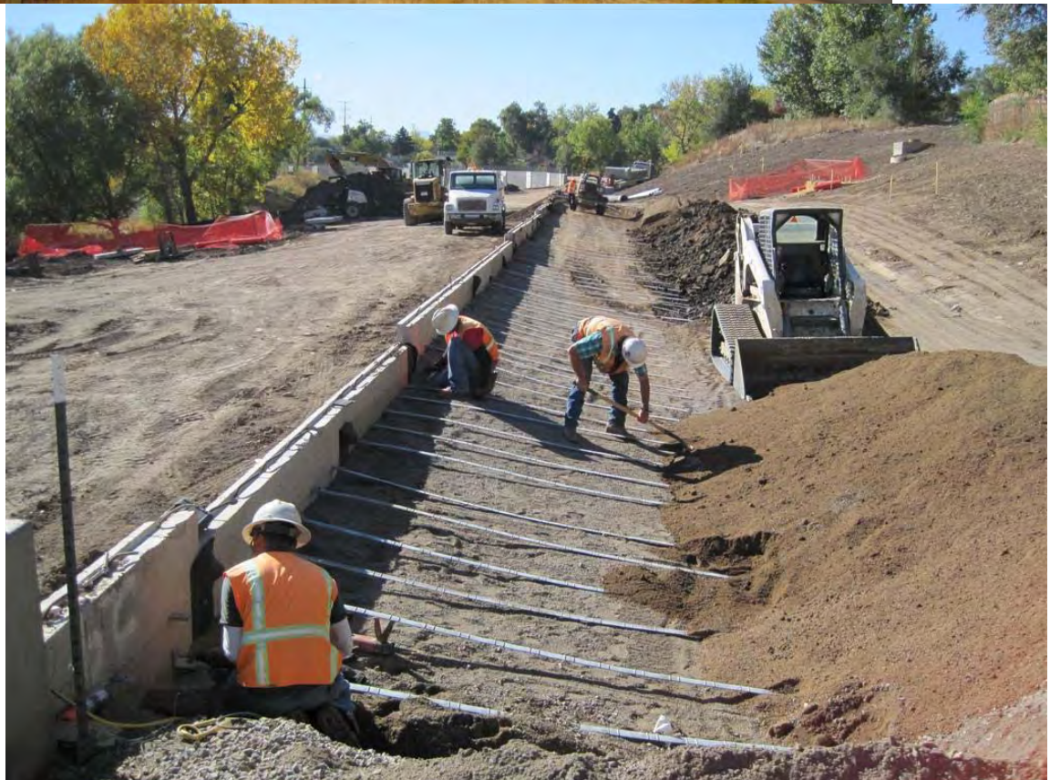
Knox Station Wall Construction
