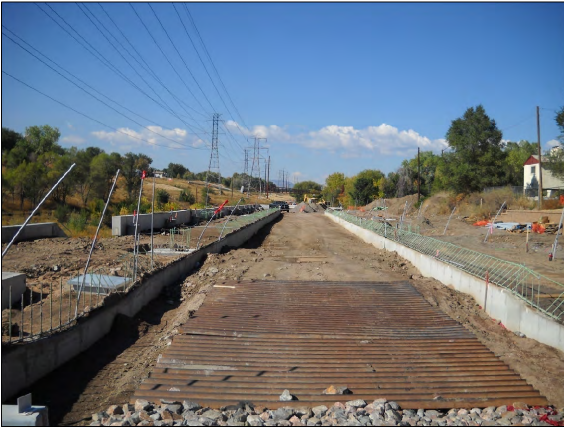
Perry Street Station foundations
