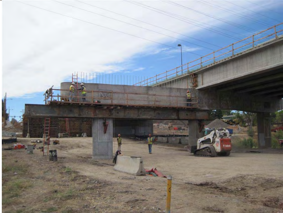
Sheridan Bridge Substructure Construction
