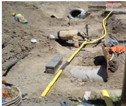
Gas Line Relocation at 13th Avenue and Dudley
