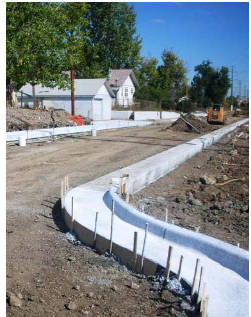
12th Avenue Curb and Gutter Work October 7, 2009
