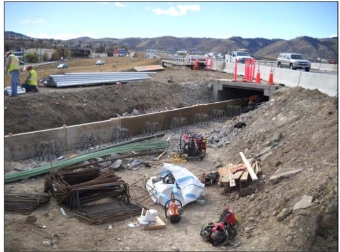
Construction on the tunnel under I-70 October 15, 2009
