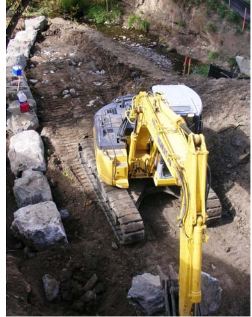
Lakewood Gulch Channel Protection October 7, 2009
