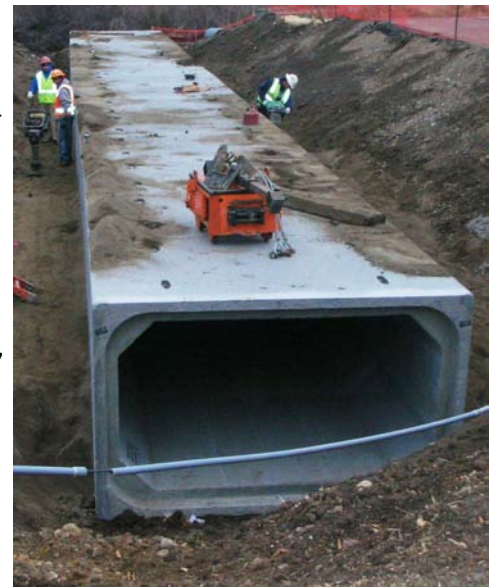
North Avenue Concrete Box Culvert October 27, 2009
