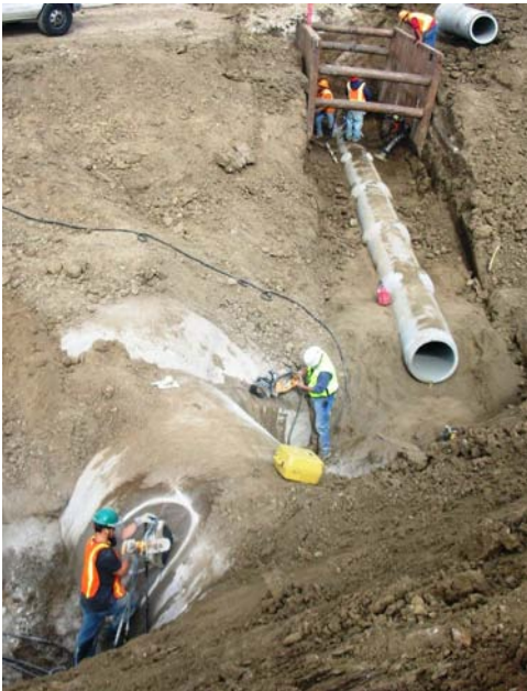
6th Avenue Storm Sewer October 7, 2009
