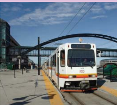
Existing Southeast Corridor Light Rail Station at Lincoln
