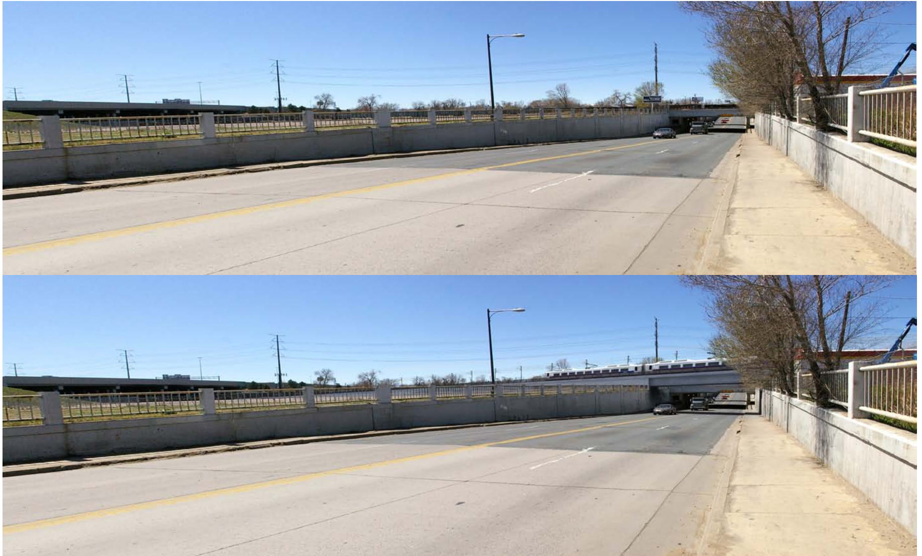
FIGURE 3.5-5. 38 TH AVENUE UNDERPASS – LOOKING WEST (BEFORE AND AFTER) (DENVER SECTION)
