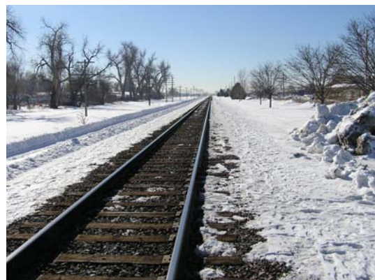
UP line south of Bridge Street (Hwy 7)
