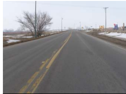
SH 2 north of 96 th Avenue
