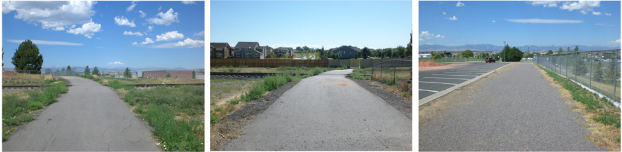
Existing Site Photos
