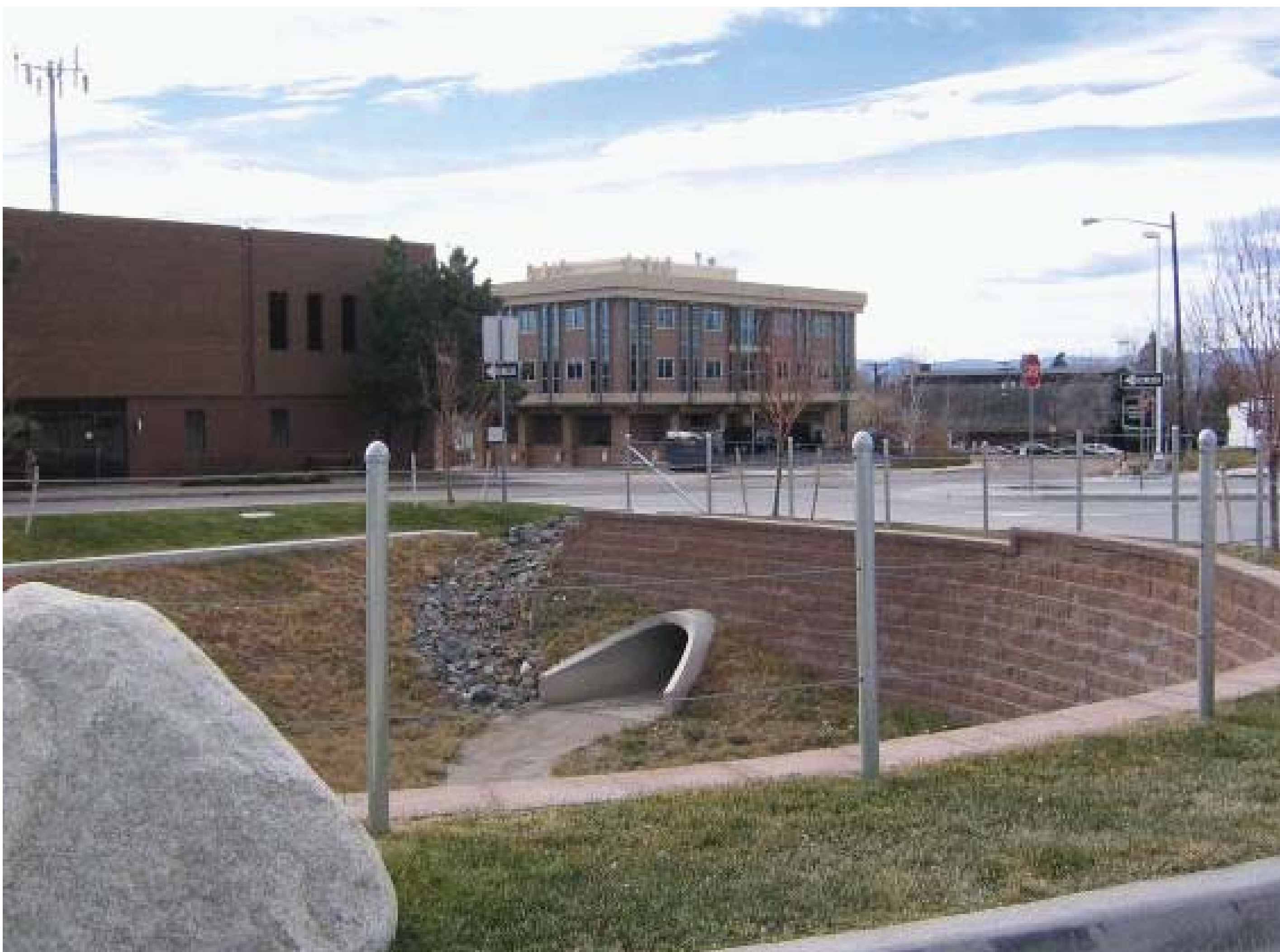
Decorative Post and Cable for visually sensitive areas (e.g. historic districts, bridges, near stations)
